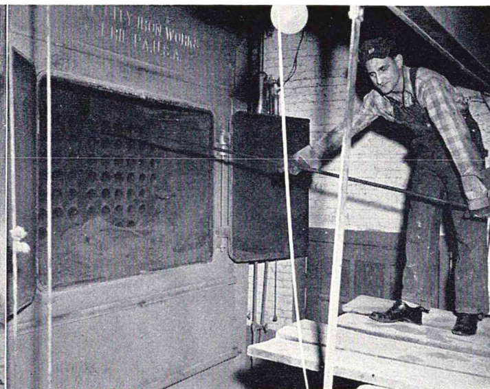
Every morning the pipes in the boilers must be cleaned out. John Trojan is doing this with a long handled brush.
